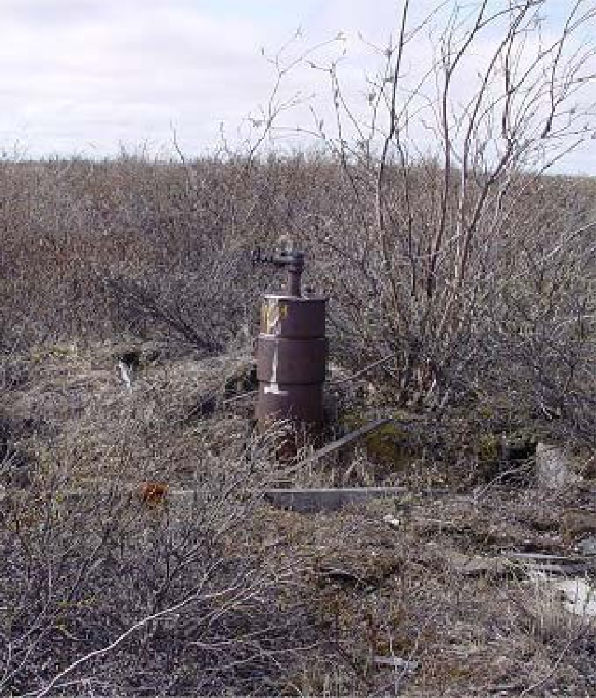
Primitive, rusting wellhead and wood debris
