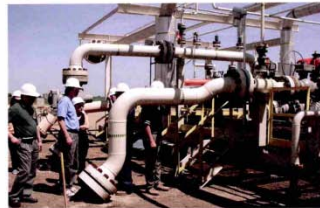
Figure 2. CO 2 is pumped 4800 feet underground at the CO 2 injection site in the Weyburn-Midale Field in Saskatchewan, Canada.
