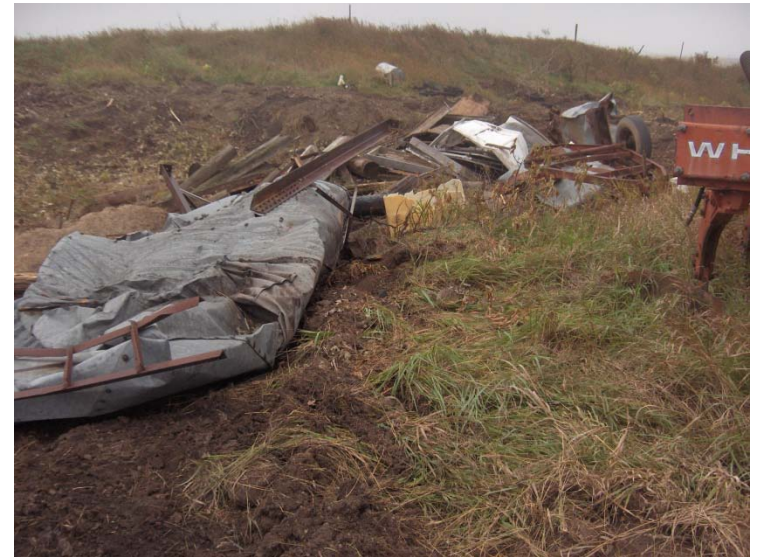
20 Cubic Yards of General Debris
