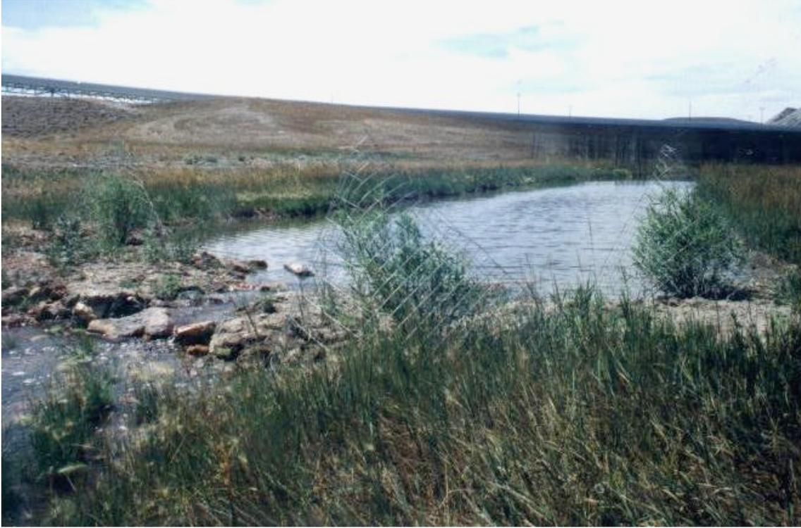
**Figure 4: Pool and Counter-Weir Sequence on Lower Section of Reclaimed Porcupine Creek Channel with Caged Coyote Willow (*Salix exigua*) Plantings**
