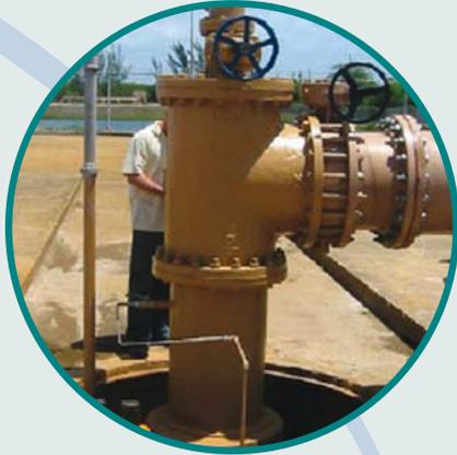
Treated municipal wastewater is pumped more than 3,000 feet deep underground through a Class I injection well in South Florida.
