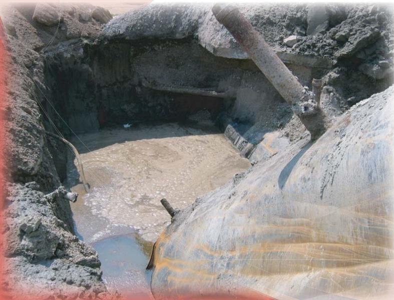
*A leaking underground storage tank is removed from gasoline-contaminated ground water.*
