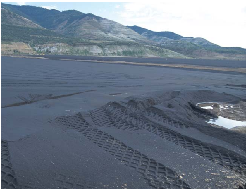
Slag placement as part of the Central Impoundment Area Repository cover system, Bunker Hill Superfund site near Kellogg, Idaho. The site is located in the silver, lead, and zinc mining district. (Image circa June 2000.)
