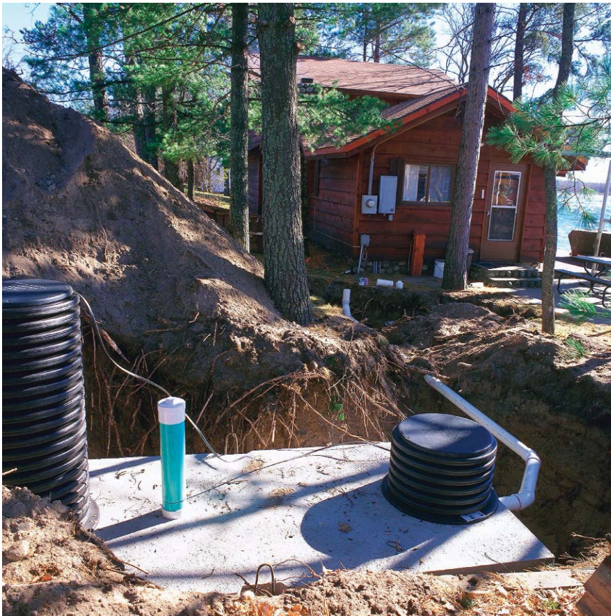
A newly installed septic tank at a lake-side cabin. The tank has been installed in a hillside, which requires tall and short access points to facilitate periodic inspection and maintenance and accommodate slope.
