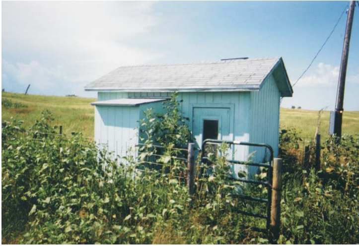
A well house for a municipal well in Tripp County, South Dakota.
