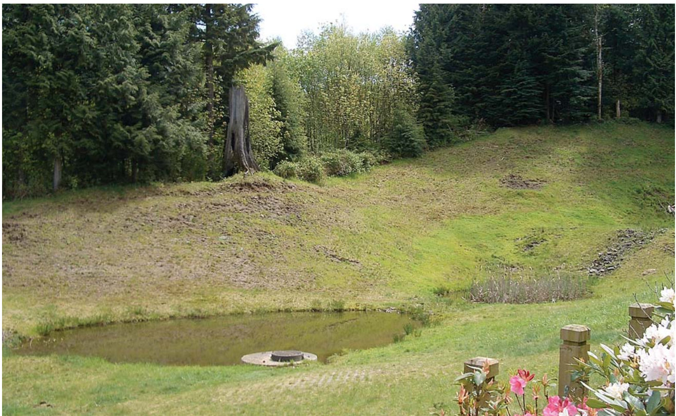
A system of stormwater infiltration ponds in the Uplands neighborhood of North Bend, Washington.
