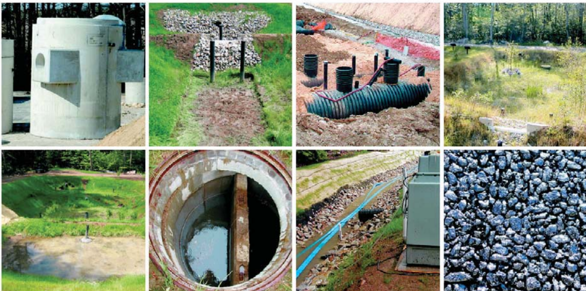
Photos: University of New Hampshire Stormwater Center
