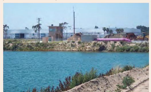
Water is then sent to groundwater recharge basins, where it ultimately becomes part of north and central Orange County's drinking water supply.
