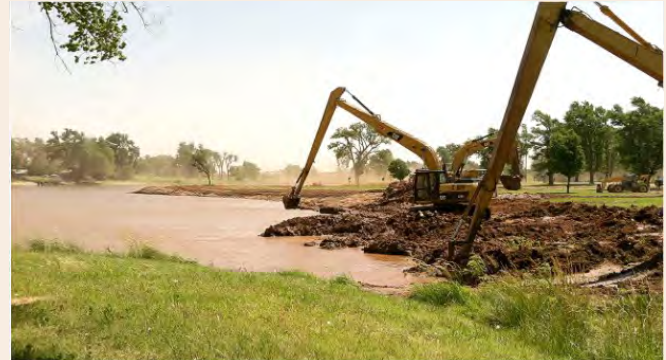
Digging to increase pond capacity on a farm in Kansas to supply water for hydraulic fracturing operations. Source – CNN Money, Blake Ellis
