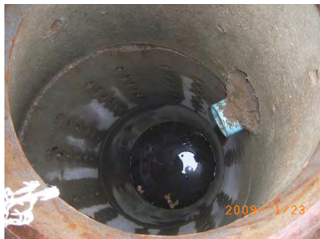
Typical dry well used to direct stormwater to the subsurface in Oregon.
