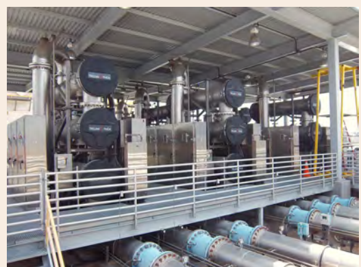
Three-step advanced treatment process consisting of microfiltration (top photo), reverse osmosis (middle photo), and ultraviolet light with hydrogen peroxide (bottom photo).
