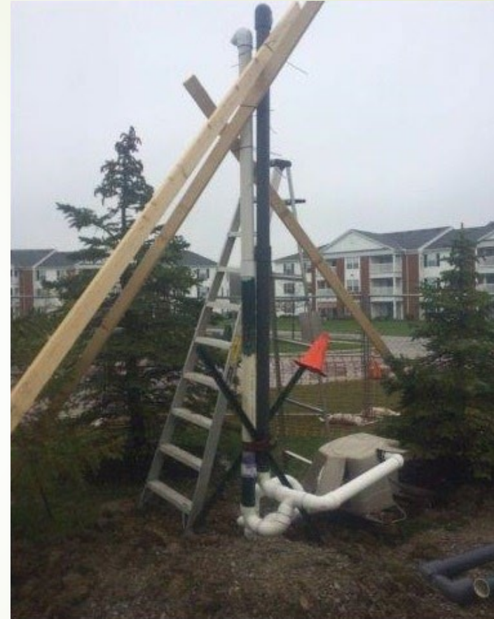
A former Clinton production well in Lorain County, Ohio, plugged in 1922 and found leaking Methane after development of an Apartment Complex. To address the leaking methane, a vent system was installed for safety purposes. The well has not been re-plugged. Source: ALL Consulting, LLC
