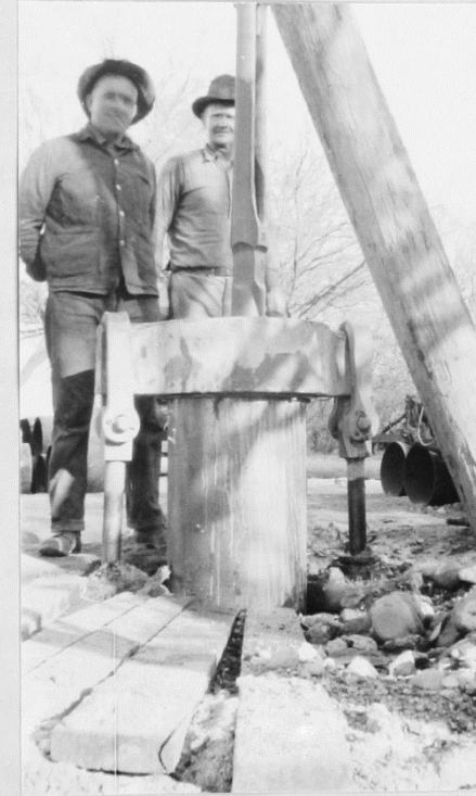
Fig. 18.- Forcing stovepipe casing down with hydraulic jacks.
