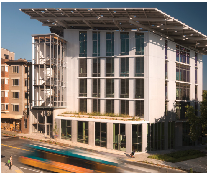
The Bullitt Center in Seattle, Washington, is the first commercial living building. It collects and treats rooftop water for potable reuse and treats greywater in a constructed wetland planter on the side of the building.
