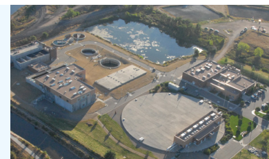
Denver Water’s Recycling Plant treats and delivers billions of gallons of water every year for industrial and outdoor irrigation uses.
