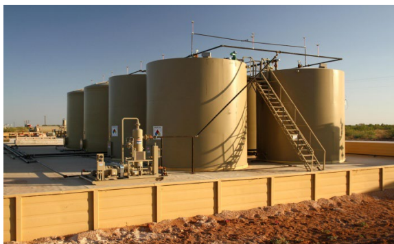
Figure 4-19 Secondary containment structure- Source, ©2014 Falcon Technologies and Services, Inc. All rights reserved.
