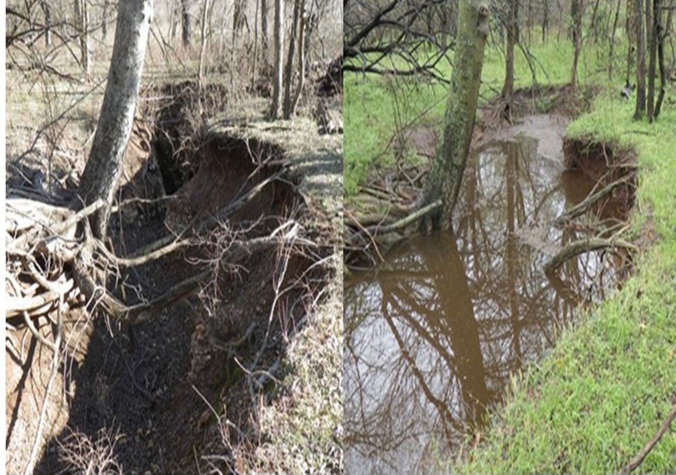
Sink hole during dry conditions
