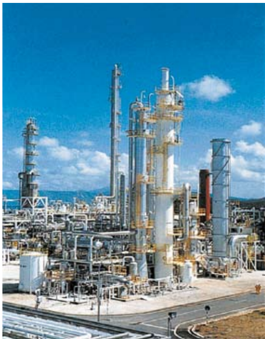
Figure 3.5 CO 2 capture plant in Malaysia using a 200 tonne d -1 KEPSCO/MHI chemical solvent process (Courtesy of Mitsubishi).
