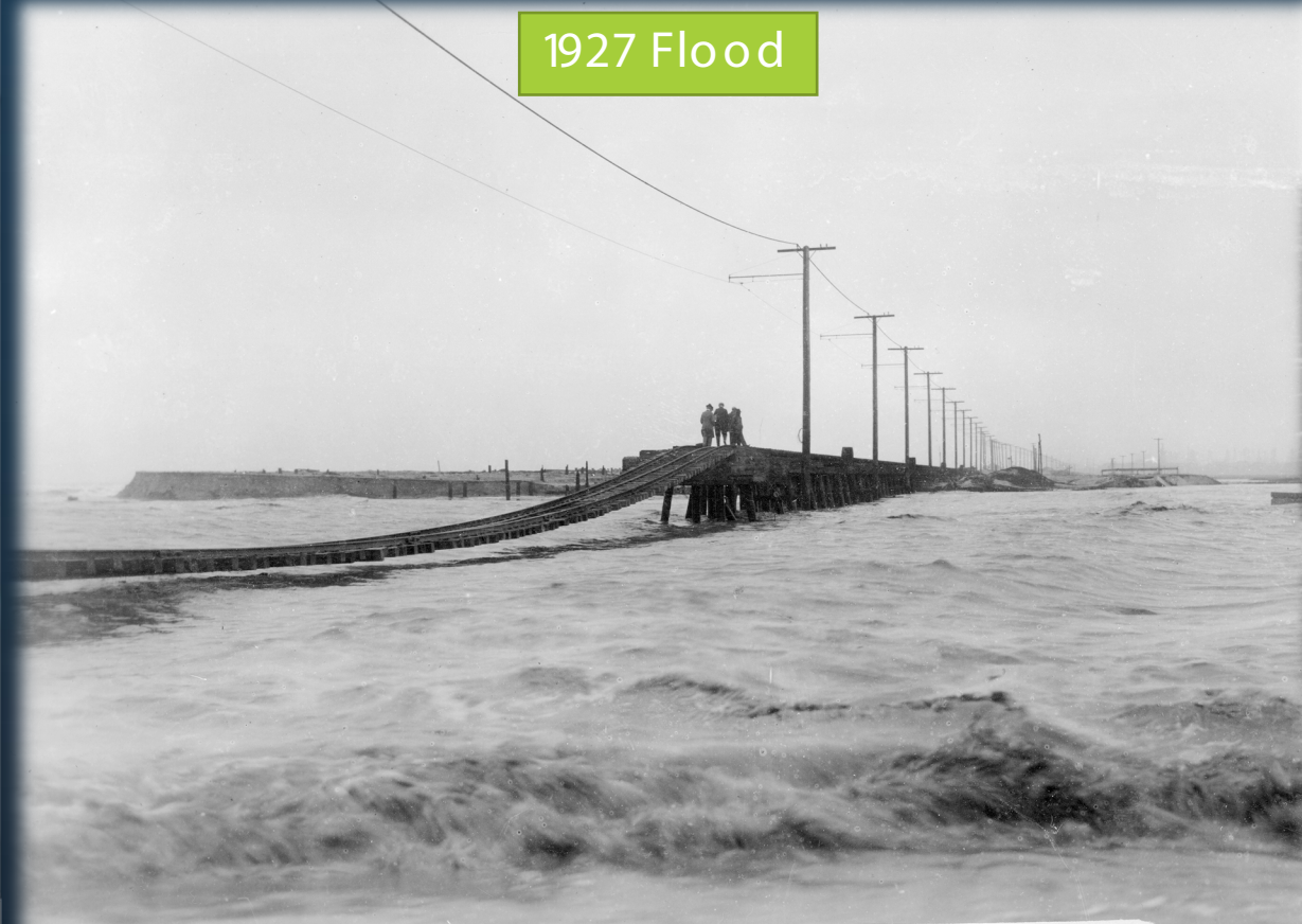
1927 FLOOD Thousand foot channel when impounded flood waters broke through to the Ocean. The Coast Blvd. & P.E. Railroad suffered extreme damage as shown.
