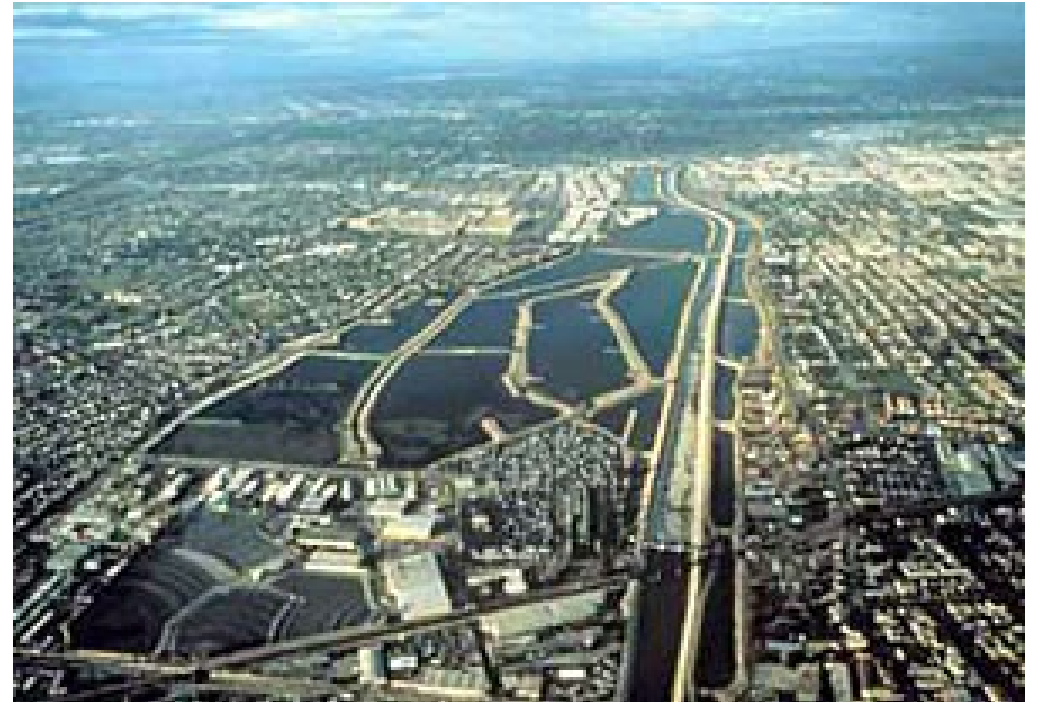
Montebello Forebay Spreading Grounds (CA): 44 MGD since 1962
